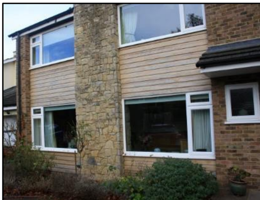
Masonry with timber cladding
