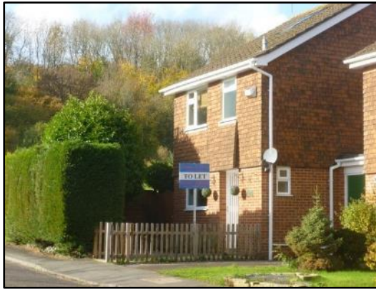
Tile hanging and brickwork
