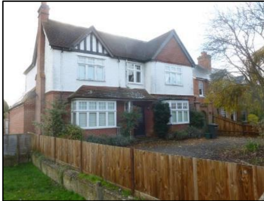
Painted render, brickwork, decorative "timbering", tile hanging
