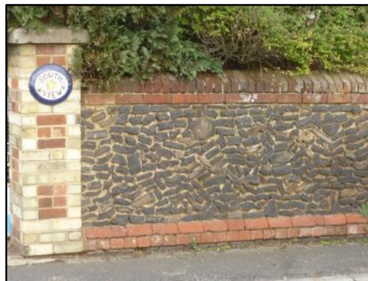
Brickwork with local Ironstone
