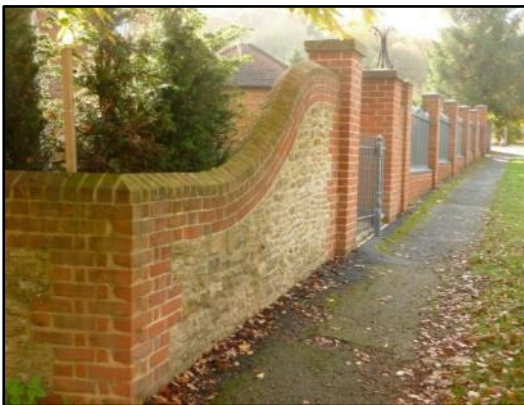
Brickwork with Bargate Stone
