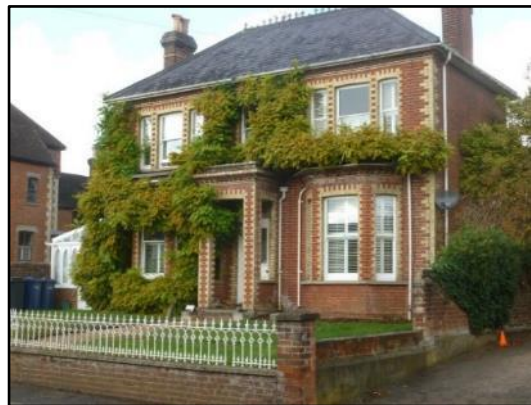
Brickwork with Metal railings
