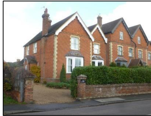
Brickwork with decorative coursing and quoins
