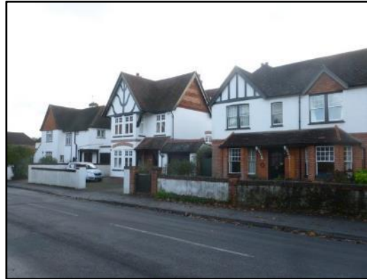
Painted render, brickwork, decorative "timbering", tile hanging
