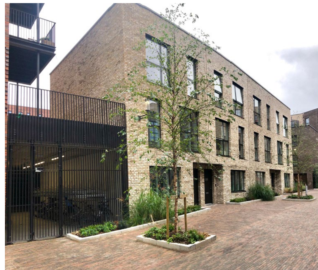
Communal cycle storage that is well-lit and has easy access to the public realm
