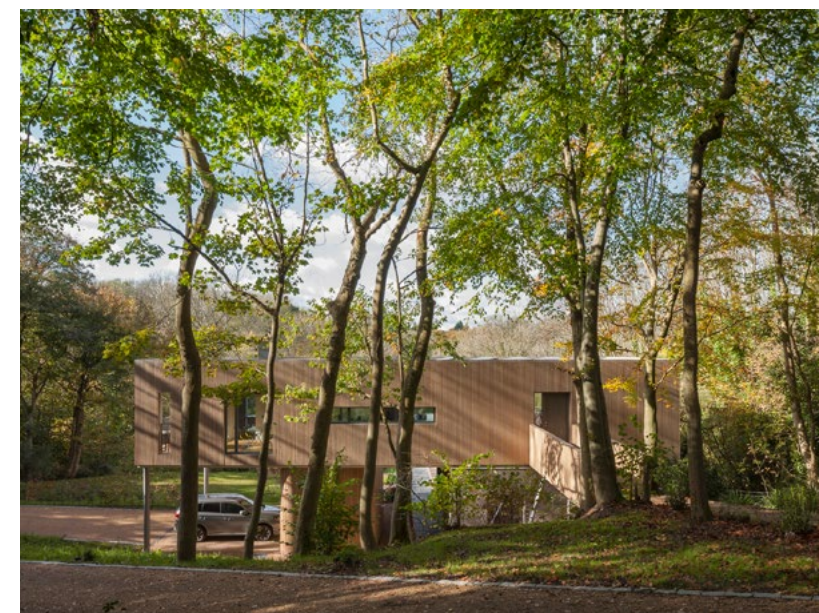
Wood House, Tatsfield by Allies and Morrison. Photo credit: ©Ståle Eriksen
