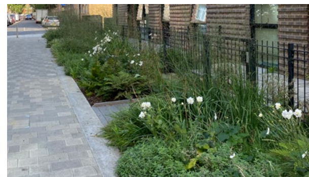
Connected rain gardens with bridges
