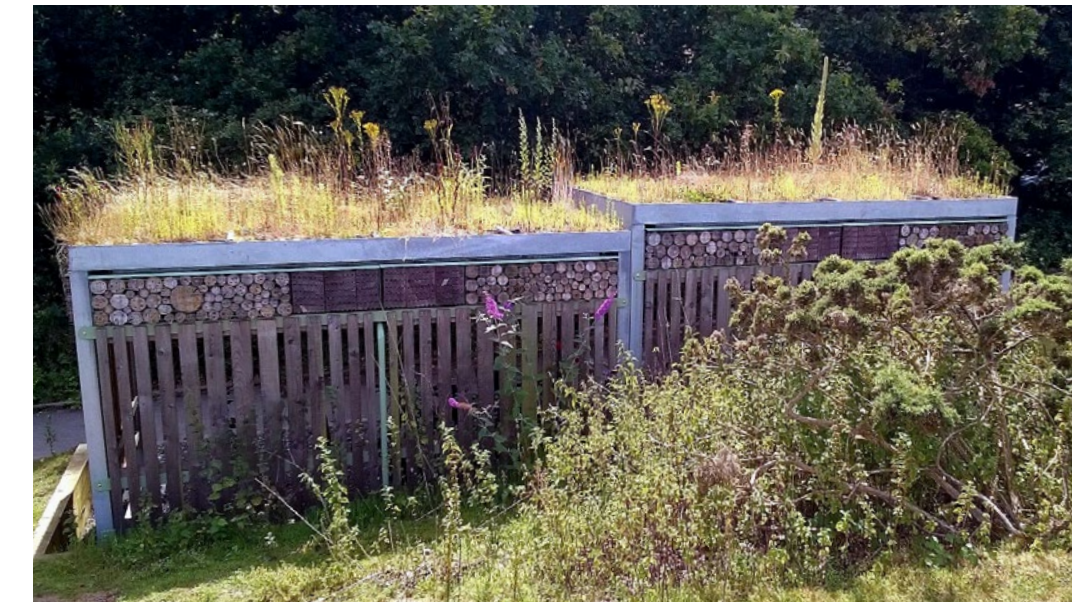
Purpose-built cycle shelter with green roof and timber cladding to blend into the surrounding landscape. Credit: Grass Roof Company
