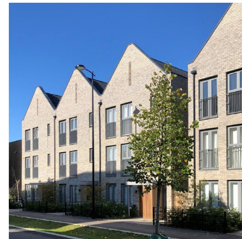
Best practice medium density housing example - Trumpington Meadows, Cambridge. Photo credit: Allies and Morrison
