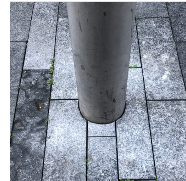
Paving cut with precision around street furniture
