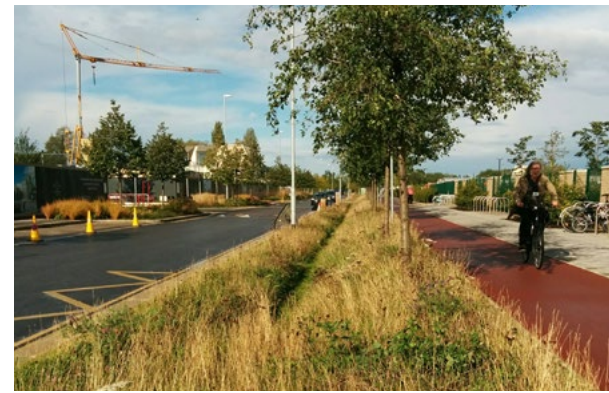
Swales and tree planting along a major street North West Cambridge, project by AECOM
