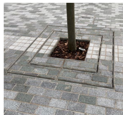
Tree grille matching to the surrounding paving
