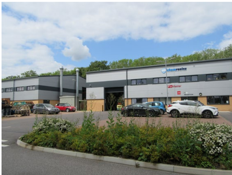
Existing business units at the Business Park
