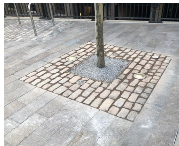
Paved tree surround with permeable surface and adequate space for growth
