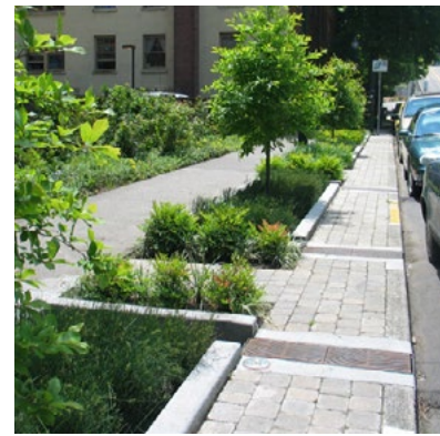
Rain gardens with drainage inlets. Credit: City of Portland
