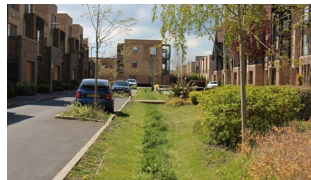
Street swale adjacent to car parking
