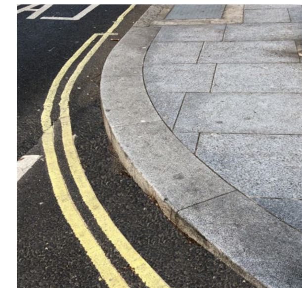
Granite kerbs will typically require less repair/replacement than concrete kerbs and will usually have a lower whole life carbon impact, when sourced sustainably
