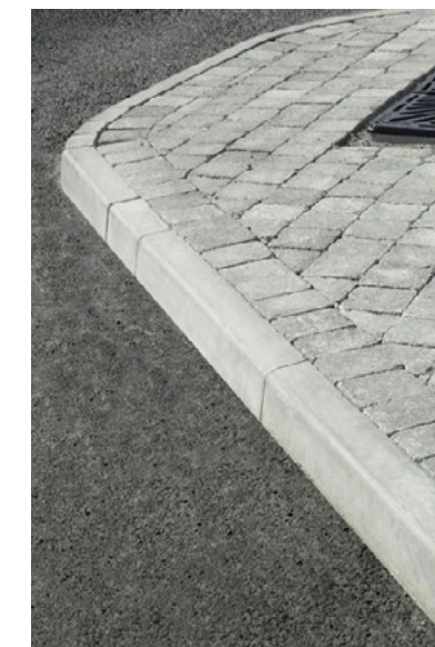
Granite kerbs will typically require less repair/replacement than concrete kerbs and will usually have a lower whole life carbon impact, when sourced sustainably
