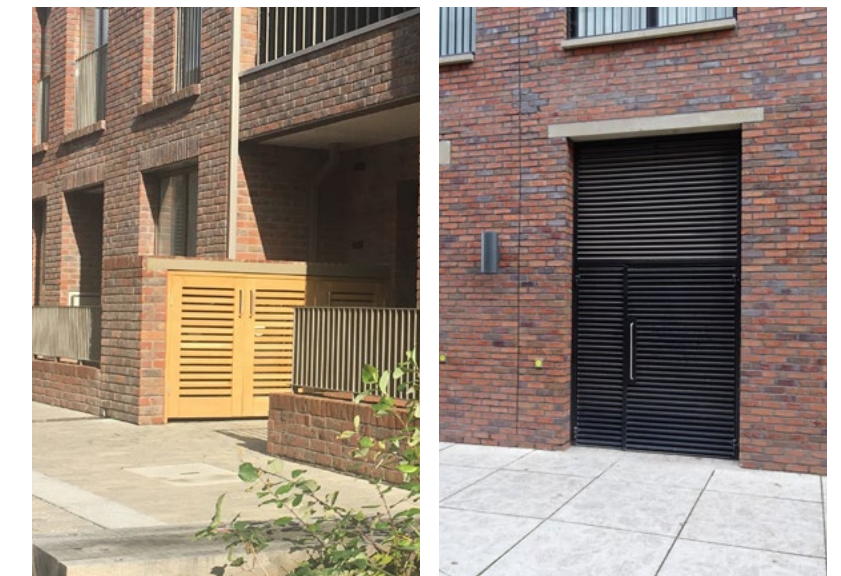
Examples of ventilated, robust waste and recycling storage integrated into the overall built form of the individual dwelling (left) and communal dwellings (right)
