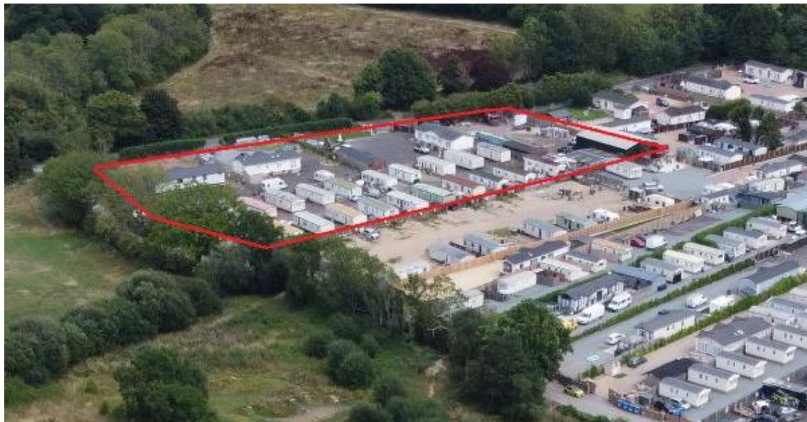
Figure 3 – drone imagery of the site captured July 2025.
