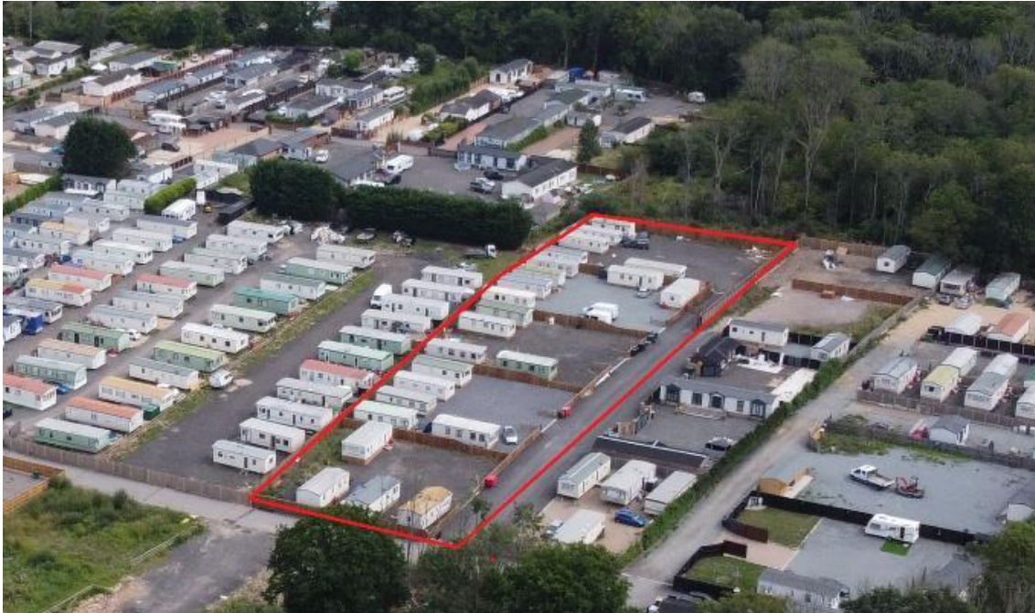
Figure 25 – drone imagery captured July 2025
