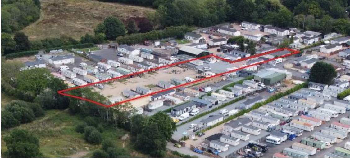
Figure 6 – drone imagery captured July 2025
