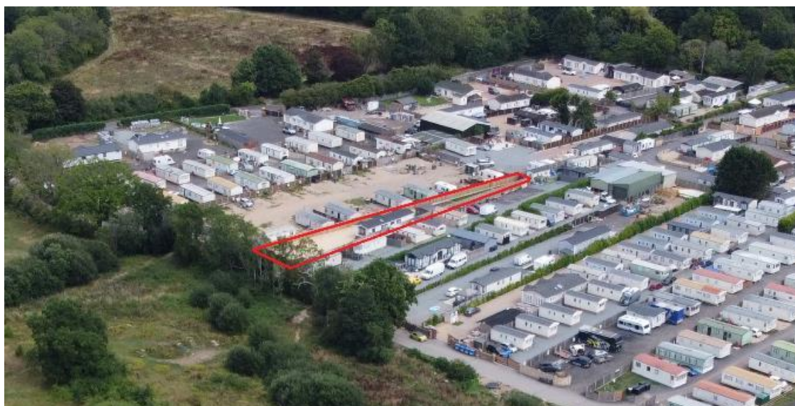
Figure 9 – drone imagery captured July 2025
