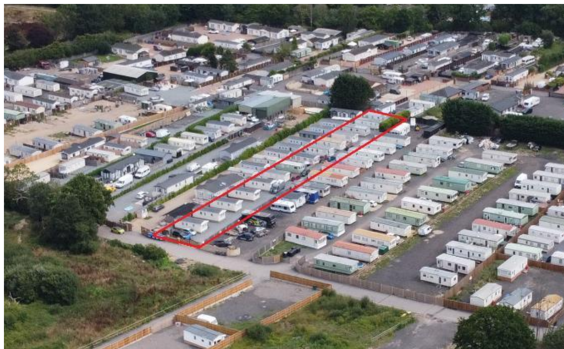
Figure 18 – Drone imagery captured July 2025
