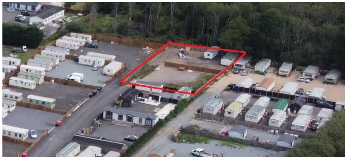
Figure 31 – drone imagery captured July 2025
