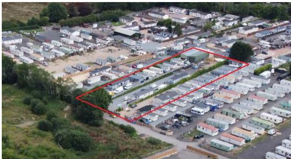
Figure 15- drone imagery captured July 2025
