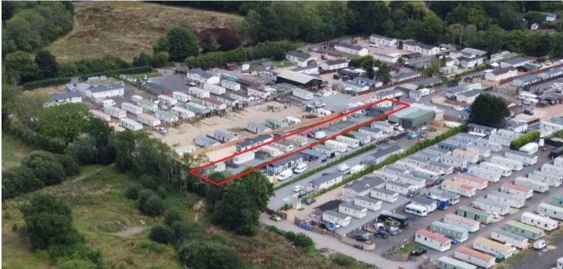
Figure 12 – drone imagery captured July 2025.
