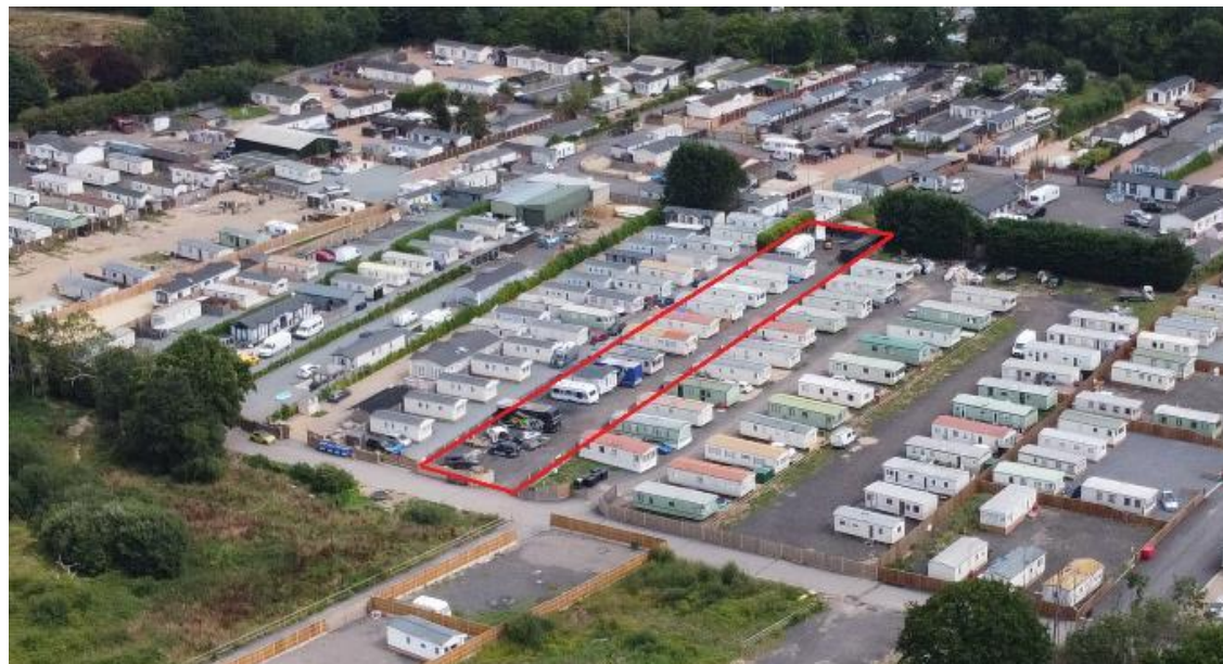
Figure 19 Drone imagery captured July 2025.
