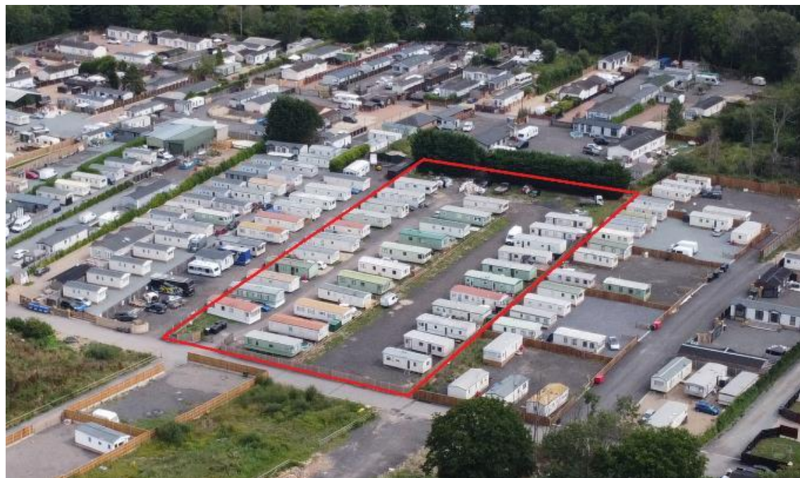
Figure 22 – drone imagery captured July 2025
