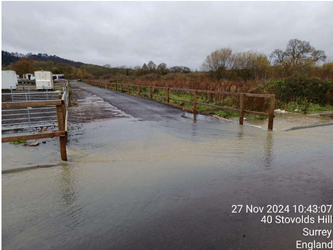
Surface water flooding at access to Plot 4.
