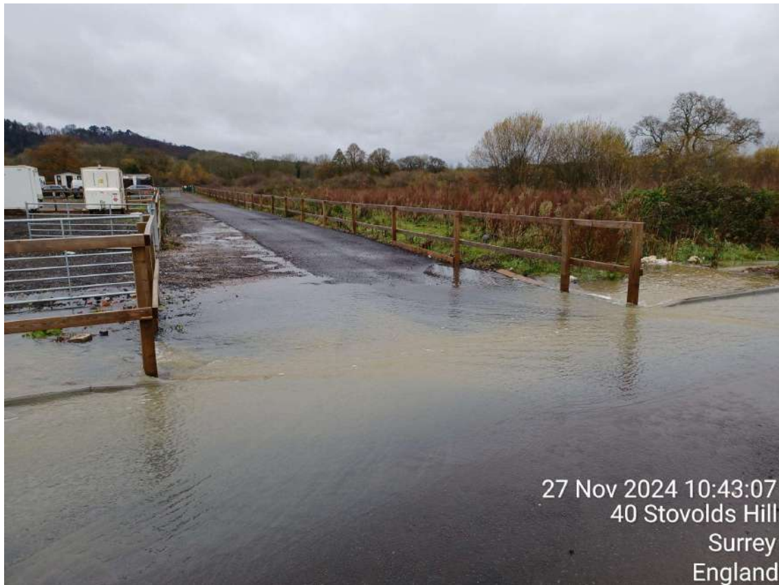
Surface water flooding at access to Plot 3.
