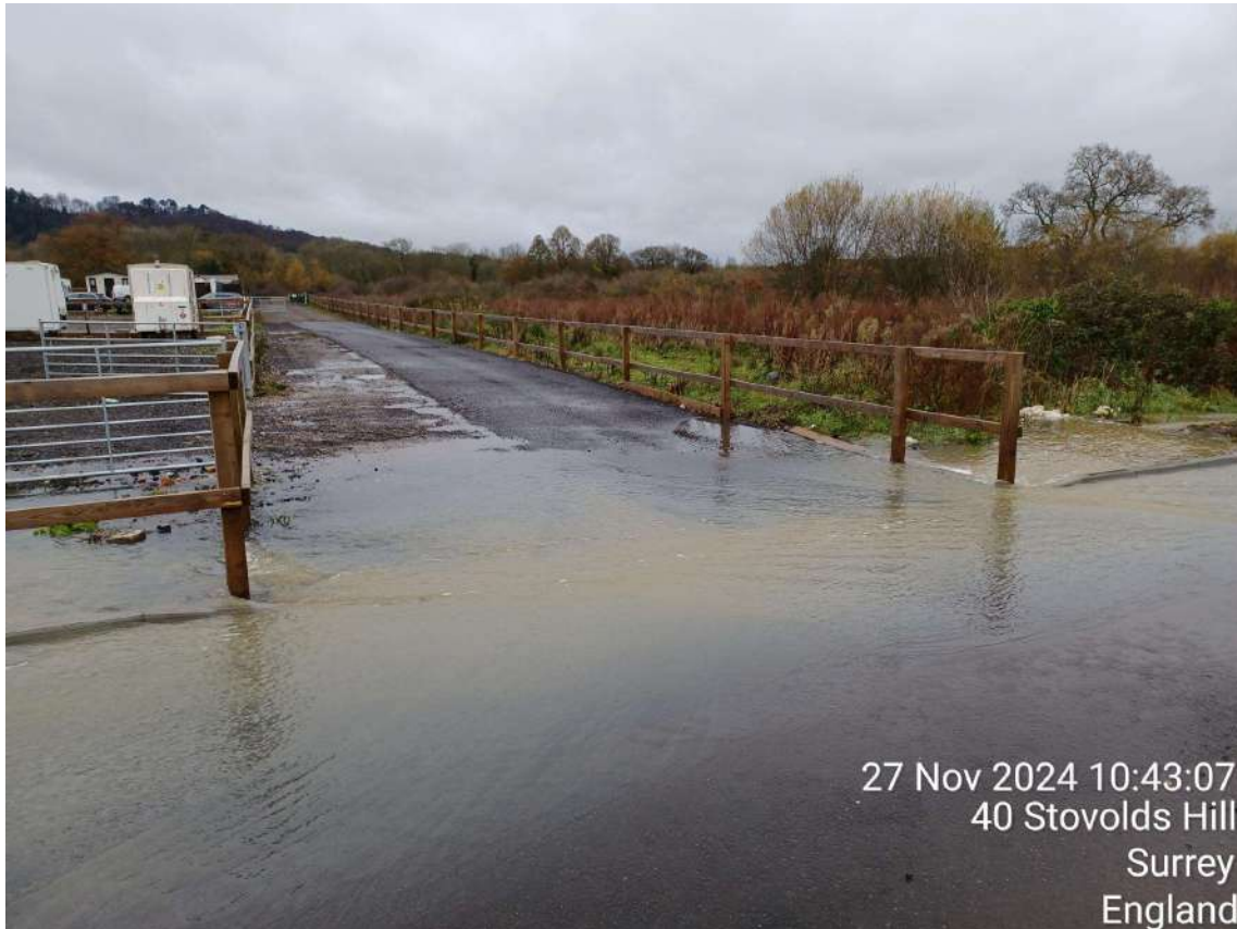
Surface water flooding at access to Plot 2.
