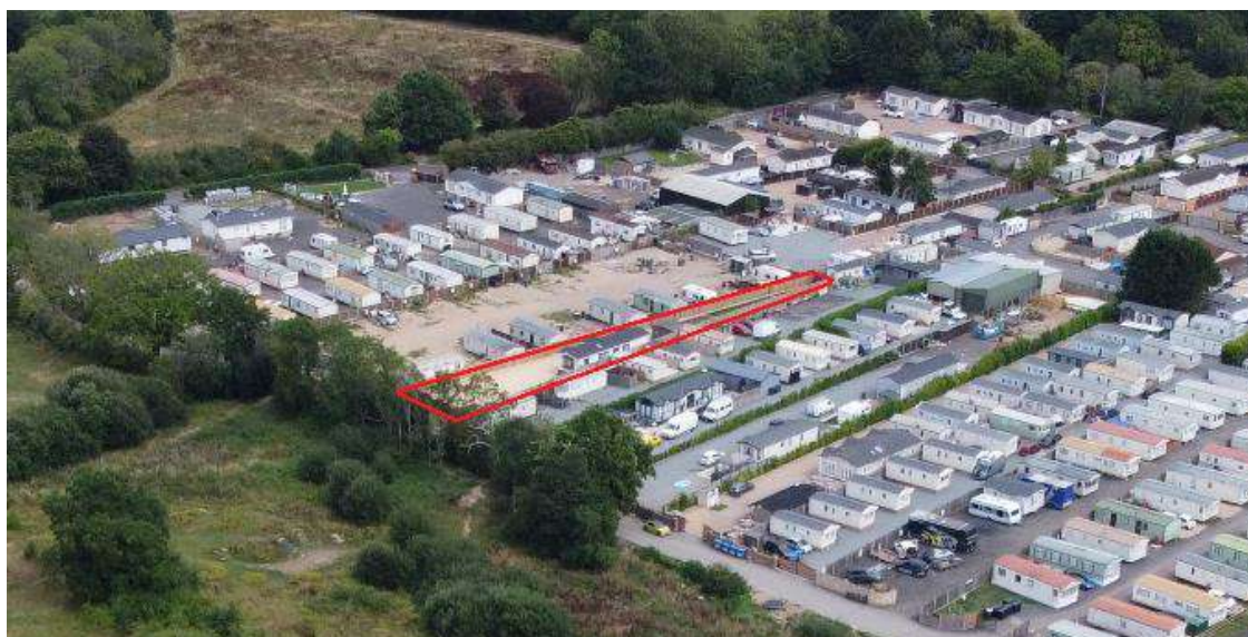
Figure 9 – drone imagery captured July 2025
