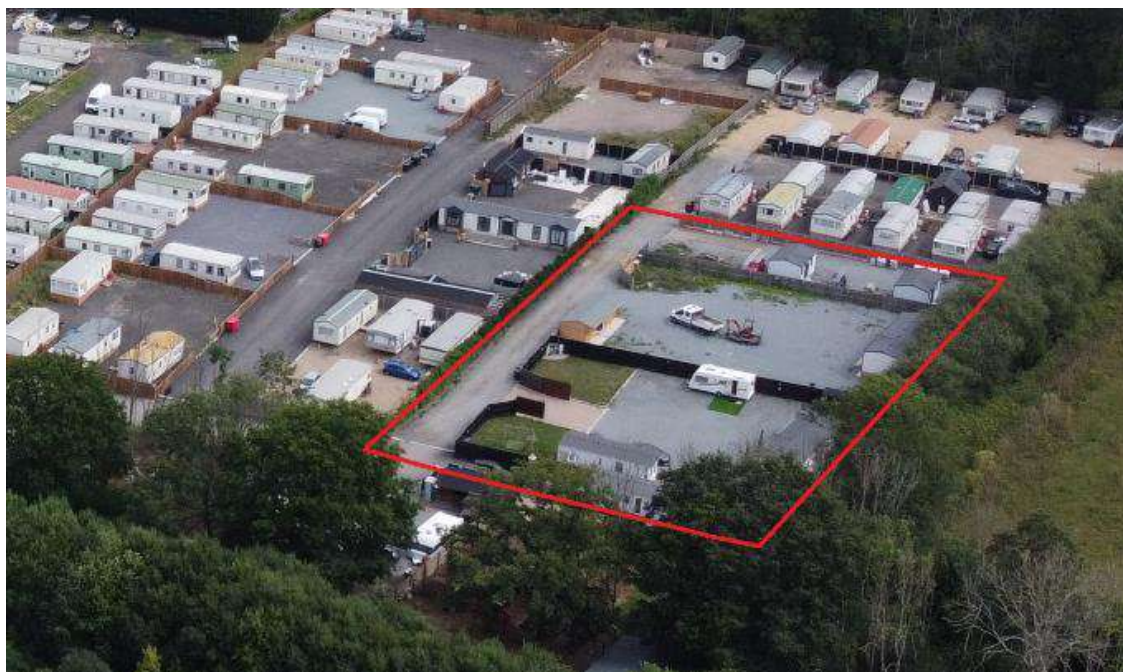
Figure 34 – Drone imagery captured July 2025
