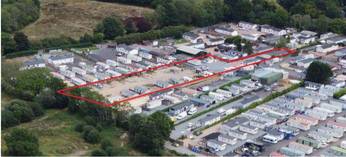
Figure 6 – drone imagery captured July 2025
