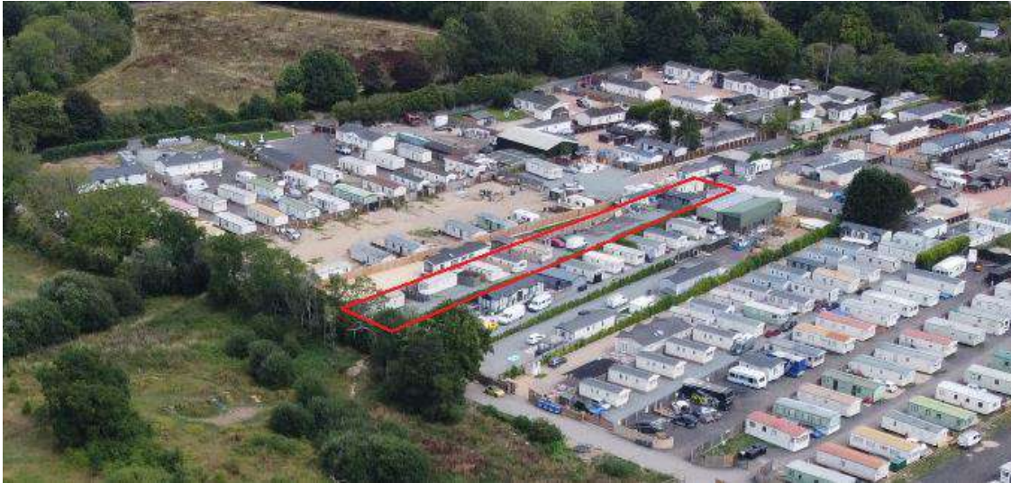
Figure 12 – drone imagery captured July 2025.
