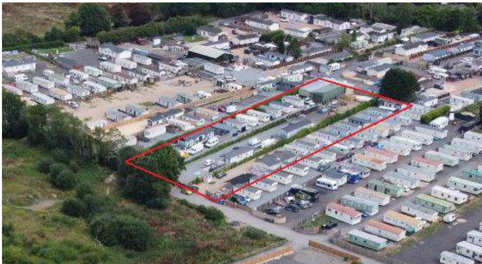
Figure 15- drone imagery captured July 2025
