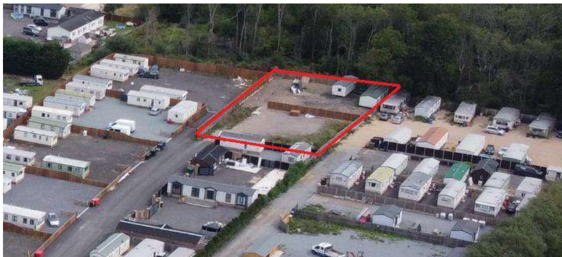
Figure 31 – drone imagery captured July 2025
