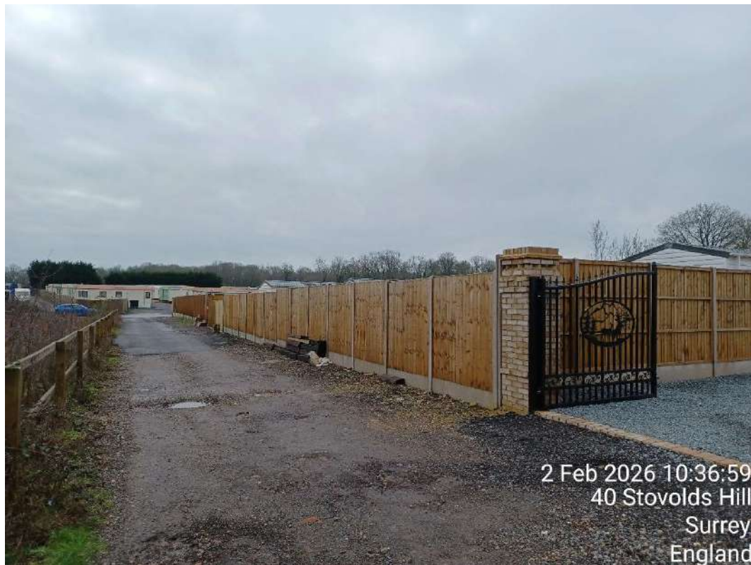
Photo 11 View south along the access drive
