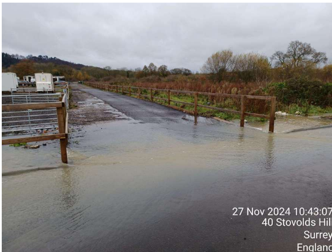
Photograph 1 – surface water flooding at access to Plot 1.
