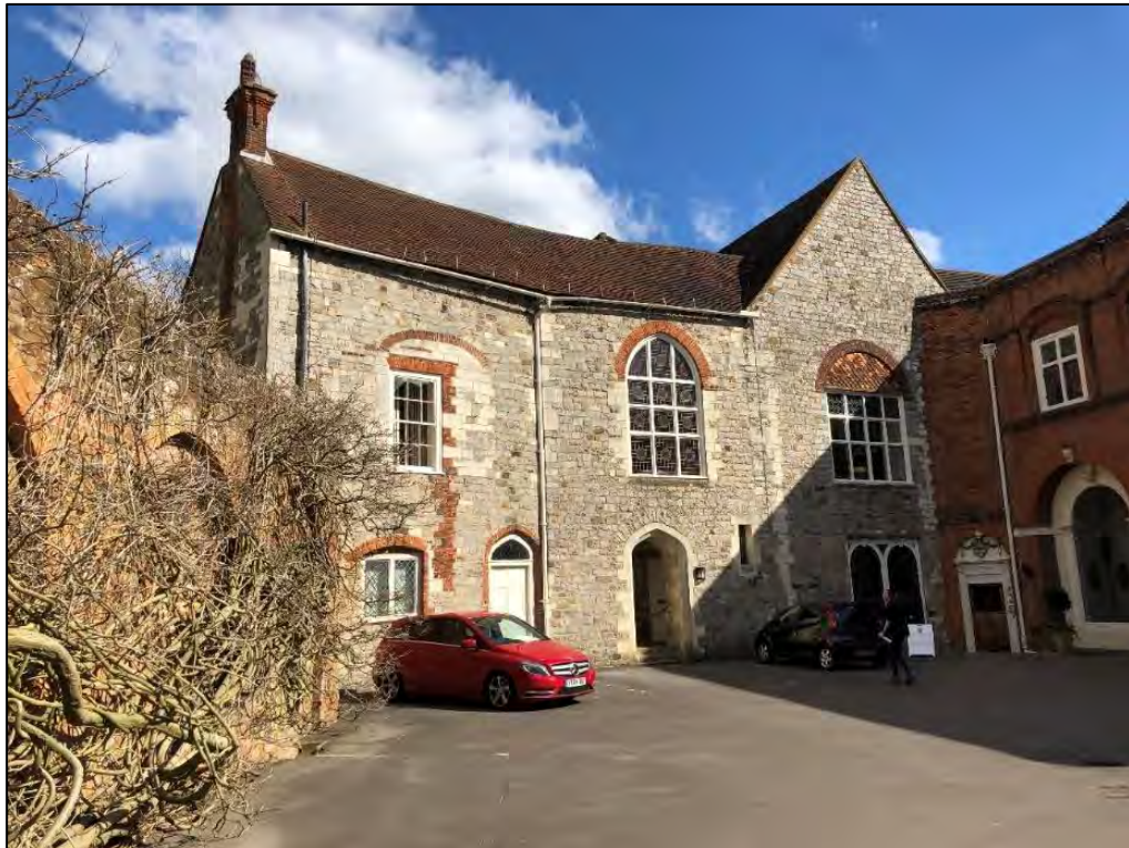
Figure 4.11: The Bishop's Chapel on the east side of the domestic courtyard.
