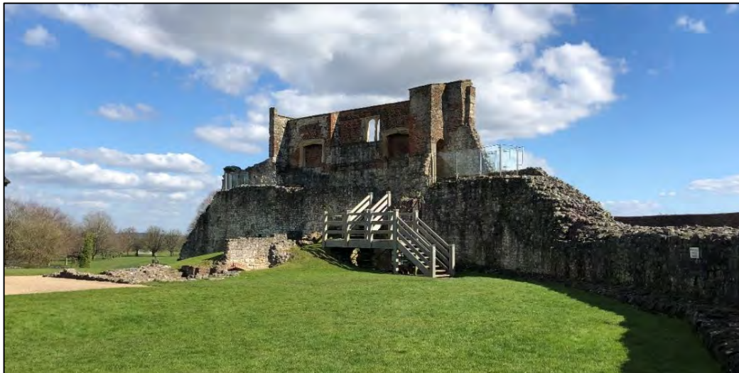
Figure 4.8: The remain of Farnham Castle Keep with later, 15 th century brickwork over the entrance.
