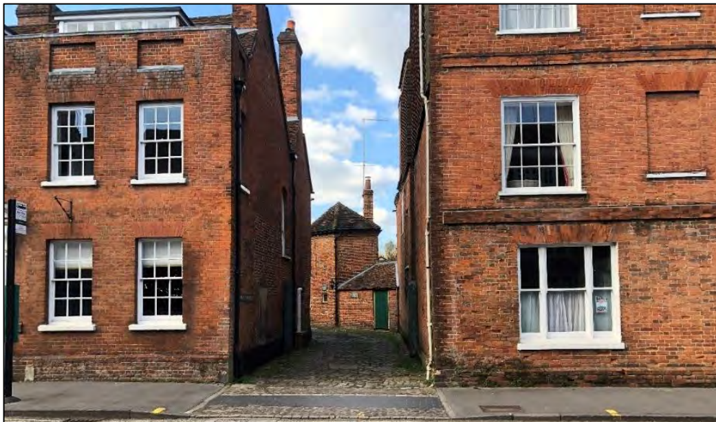
Figure 4.24: View north from West Street looking up Malthouse Yard
