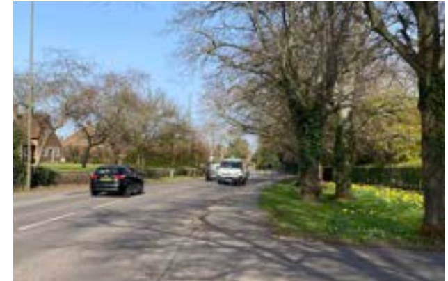
Figure 67. Constraints along West Street (e.g., third party land, mature trees) will require further investigation during the next stage of scheme development to assess the feasibility of widening the footway to provide a shared-use path (item #2)
