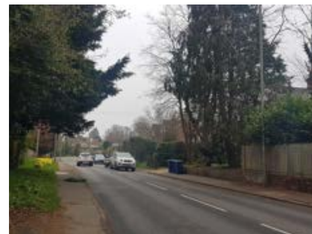
Figure 90. Narrow footways along Firgrove Hill
