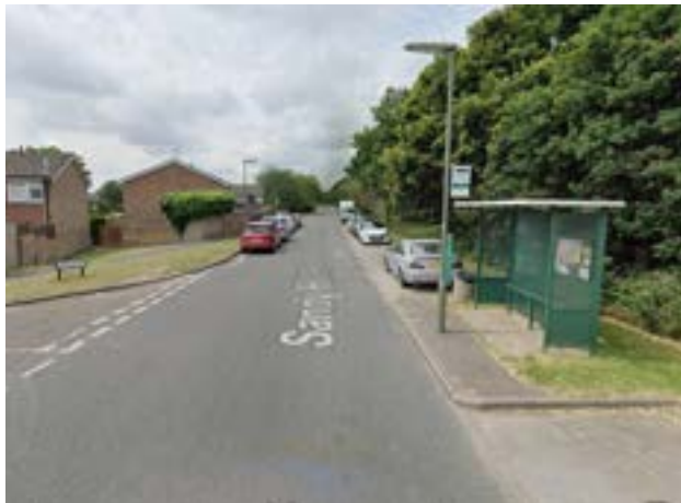
Figure 94. Poor accessibility to the bus stop infrastructures along Sandy Hill. Source: Google Street View
