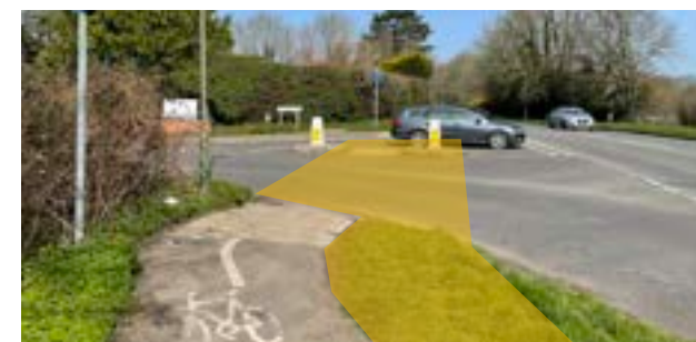
Figure 75. Weybourne Road at Monkton Lane - proposed path widening to provide segregated two-way cycle track and footway, and raised table for cycle priority at side road junctions (proposal #2; highlighted in orange) [source: Google Streetview]
