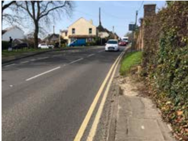
Figure 93. Lack of footway continuity along Upper Hale Road
