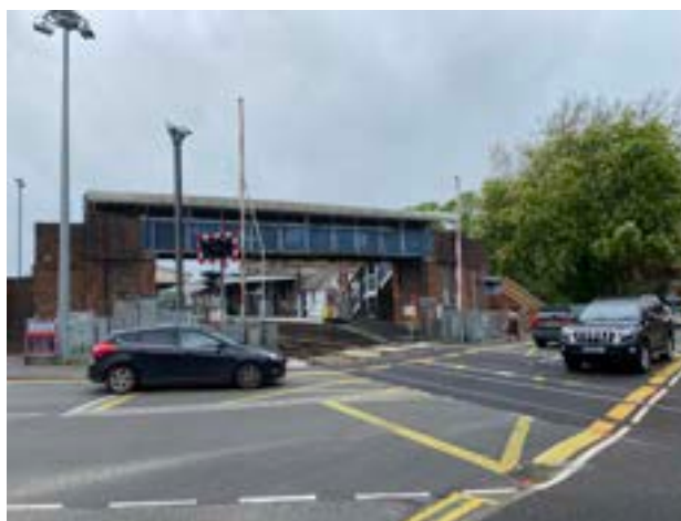
Figure 86. Level crossing at the railway station with poor pedestrian provision
