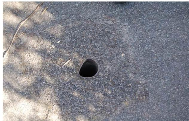
*Figure 14: Photograph of identified issue: hole in pavement*
