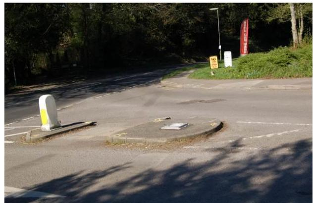
*Figure 15: Photograph of identified issue: missing internally illuminated bollard on the pedestrian refuge island, which has now been replaced*
